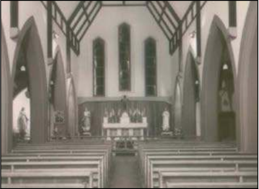
Fig. 18: St Stephen's interior received many significant improvements in the early 1950s.
