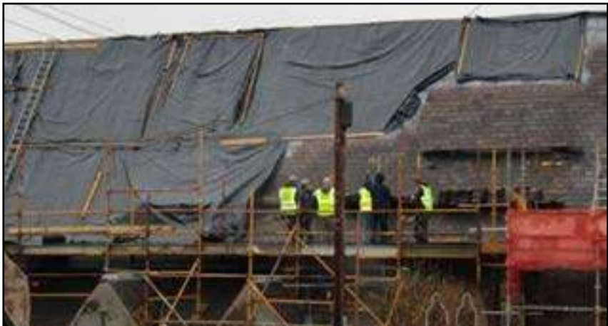
Fig. 21: Restoration work underway on the roof of St Stephen's.
