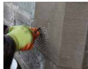
Tooling of window dressing on John Street gable.
