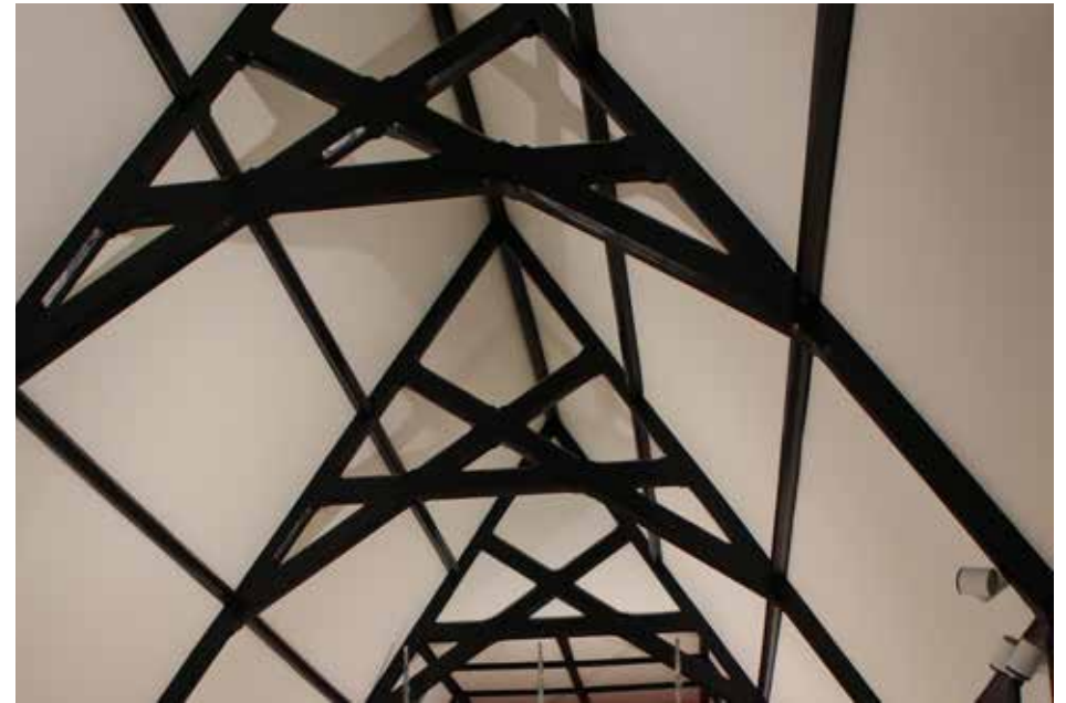
Completed knave ceiling.
