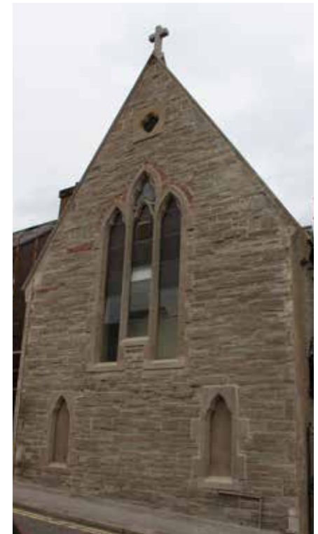
John Street gable following masonry repair.
