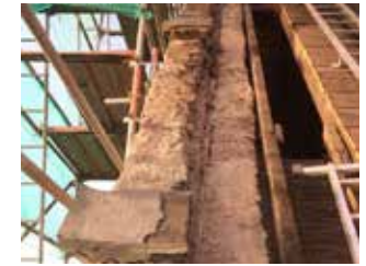
Skew stones removed from John Street gable.
