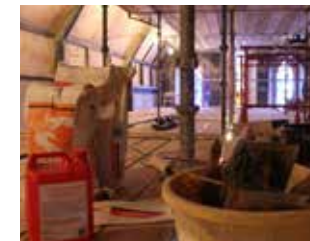
Plaster repairs being processed to knave ceiling.
