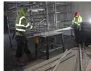
Preparation of replacement studs for installation on Sanctuary gable.
