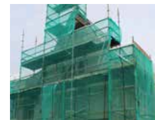
John Street gable shrouded in scaffold to enable masonry repairs.
