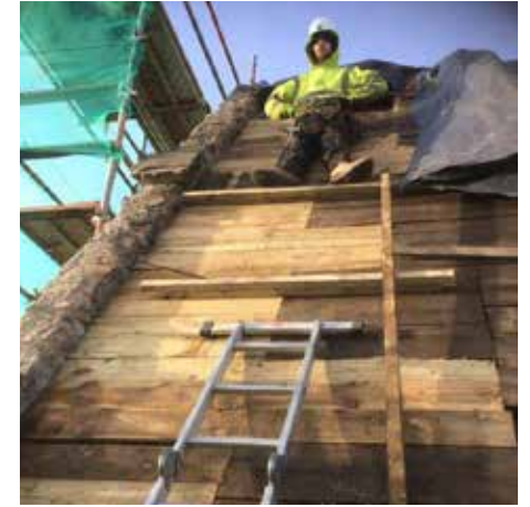
Timber roof repairs nearing completion at John St gable wall head.
