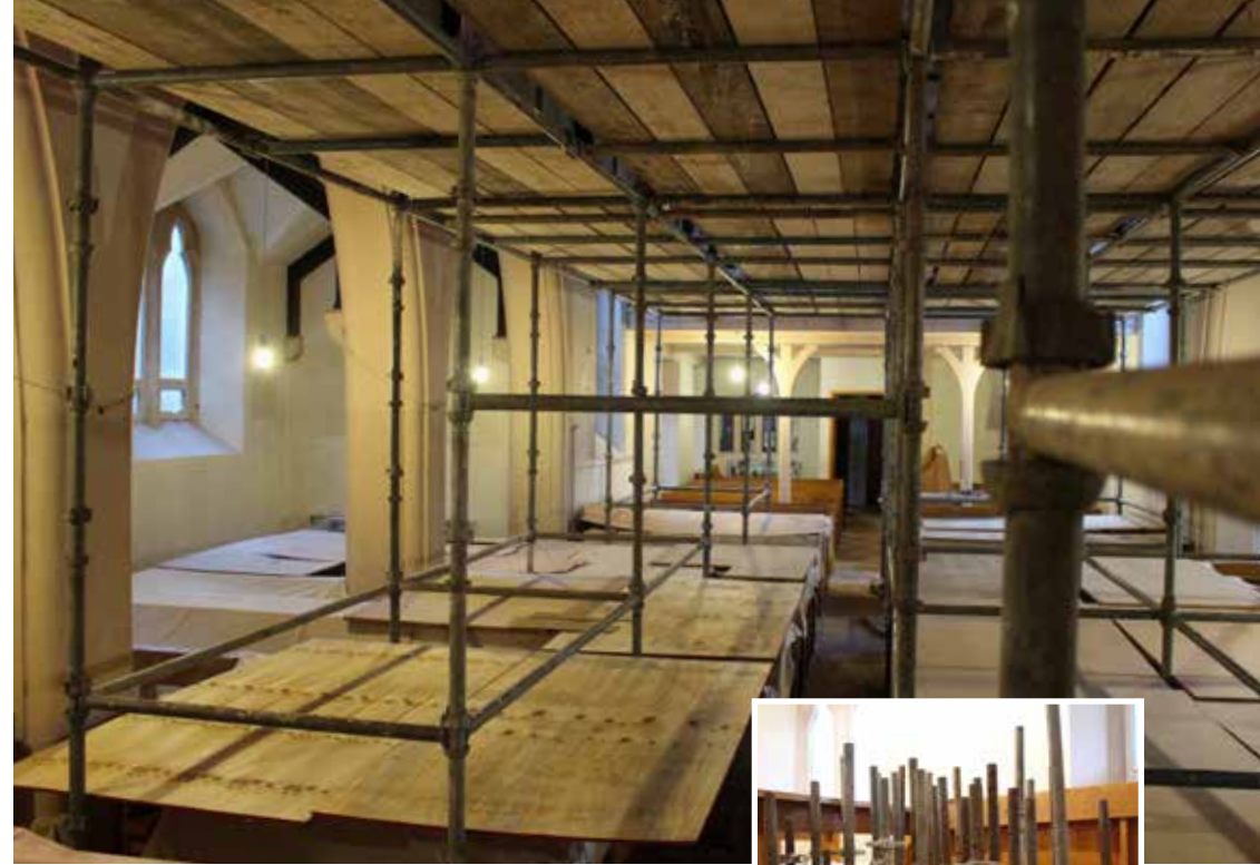
Internal scaffold to access high level knave ceiling.
