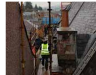
Chimney and roof repairs in progress.
