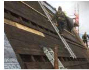
Timber roof repairs in progress.
