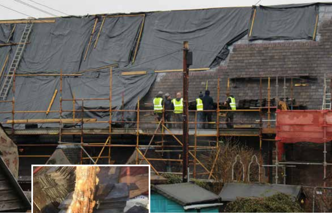
Stripping and re-slating of principal elevation.
