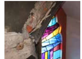
Intrusive invasion to assess fabric condition.
